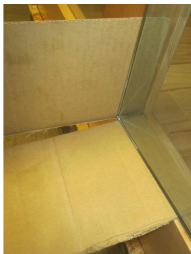
Cardboard placed vertically & horizontally between glass door and door jamb
