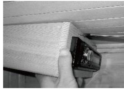
FIG-17 Screwing in the Radio Wood Housing
