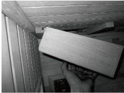
FIG-16 Installing the Radio Wood Housing
