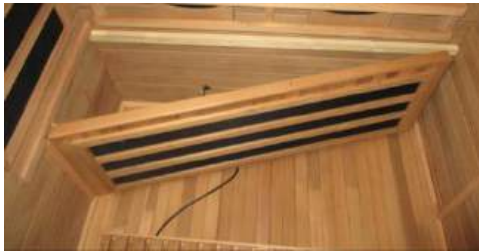
FIG-9 Installing Bench Heater
